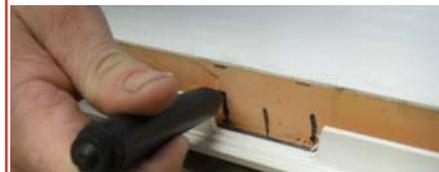
Remove cassette from the aperture and present the base clip centrally over the marks, with the up-stand positioned to the external door skin and pilot holes for the clip feet. Position using a small pin or plastic head hammer ensuring the external feet straddle the door inner and outer GRP skins, seated positively. Then introduce the secondary clips with the internal feet passing through the slots in the base clip into foam and the long external foot locating on the outside of the skin face.
