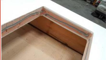
Then apply the intumescent strip starting at the base, central clip position, working your way around the aperture ensuring the intumescent sits neat, flush and central to the core, and overlaps at meeting point.
