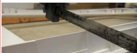
Then using a hack saw cut vertically down either side to meet the base line and carefully remove using pliers.
