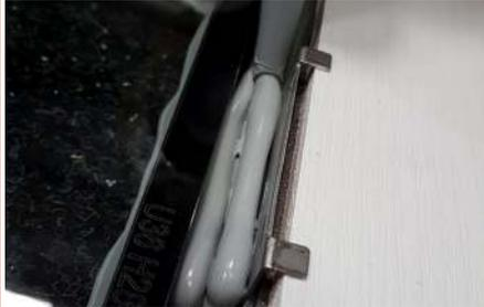
Introduce the secondary fire glass retention steel clip, make certain that the long external foot is positioned over the outside of the internal skin and persuade it into position using a small pin or plastic head hammer.
